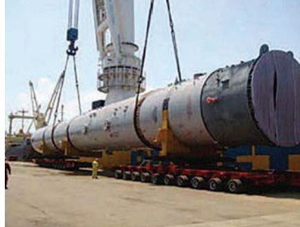
A tandem lift compensates for an off-centre CoG.
