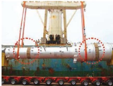
A single crane lifts a column horizontally. The position of the slings here, offset from wooden battens, indicate an off-centre CoG.
